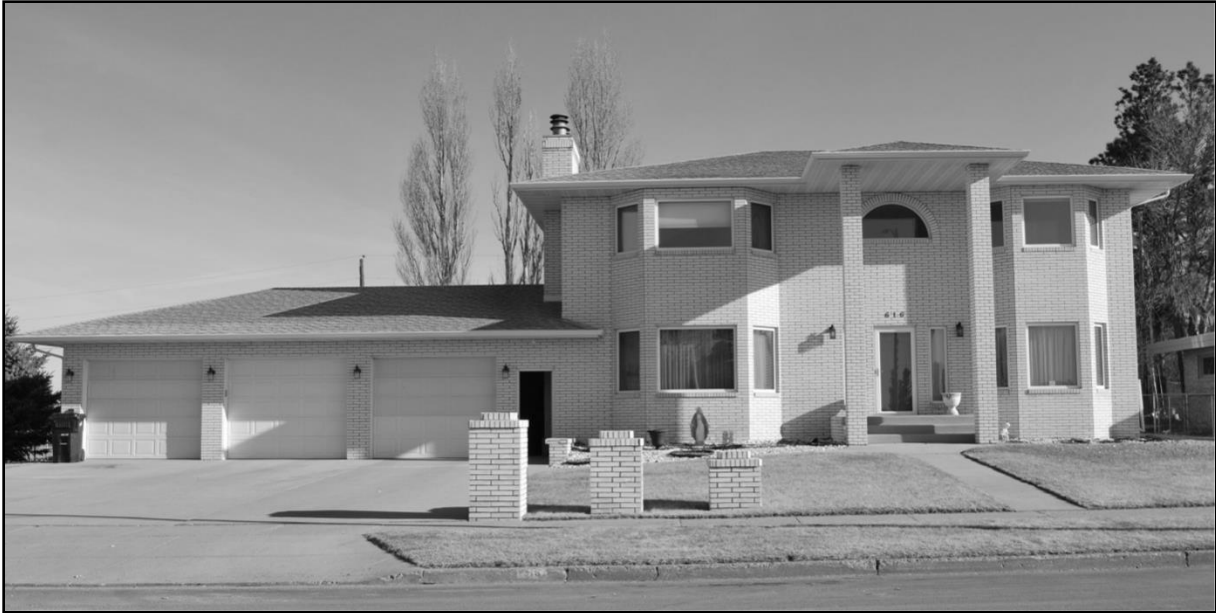
Millennium Mansion, 616 West Avenue F, Bismarck
