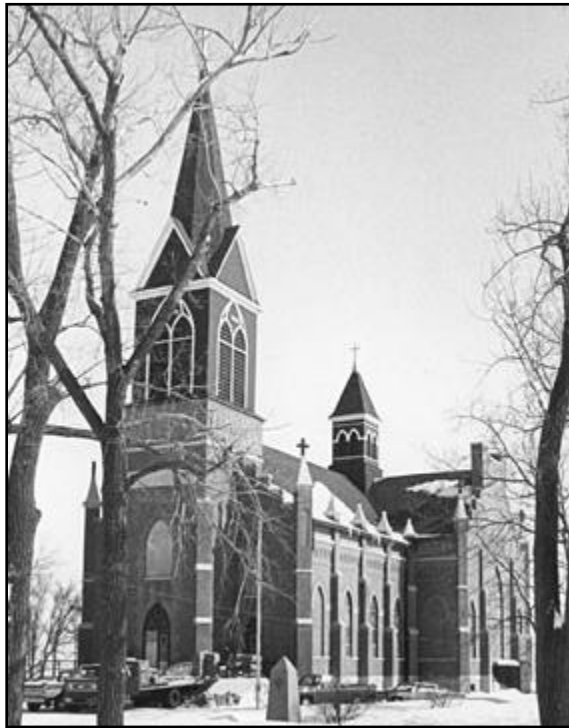
Gothic Revival Style, 32WA2
